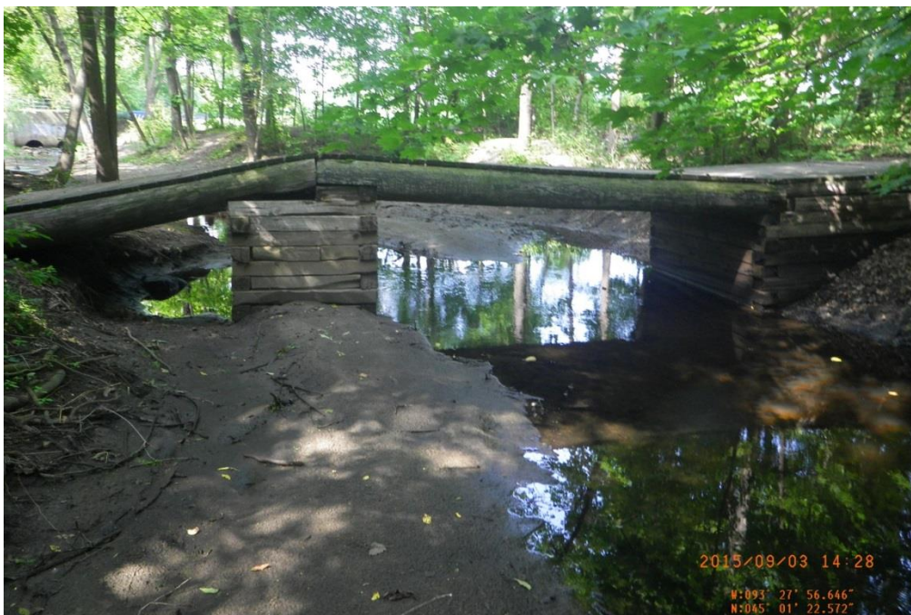
Photo 6. Site 6. Erosion around bridge abutments
