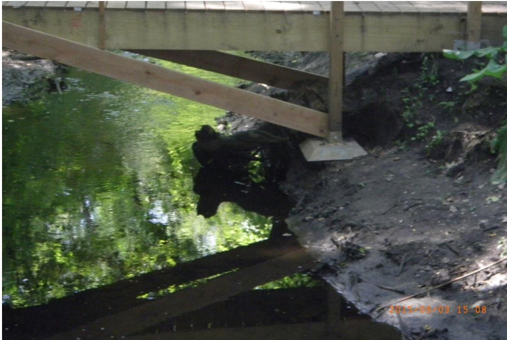
Photo 8. Site 9. Erosion around bridge abutments
