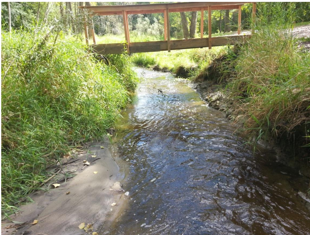
Photo 8. Site 9. Erosion around bridge abutments
