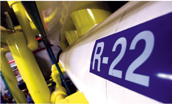
The coolant R22 is being phased out of production. An ammonia system will replace the current R22 system at PIC.
