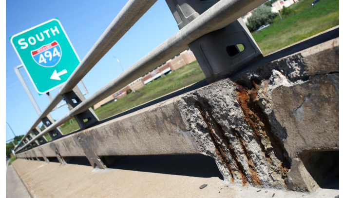
Crumbling concrete and rusty rebar can be seen on both the surface and underside of the 52-year-old bridge.
