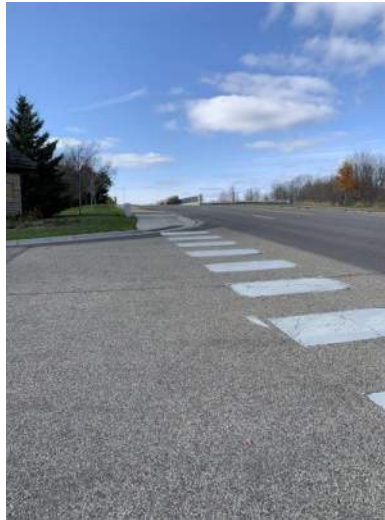
Picture 5 – Looking West (At Stop Bar)
