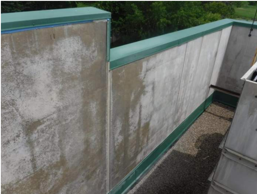
Precast discoloration observed adjacent to cooling tower
