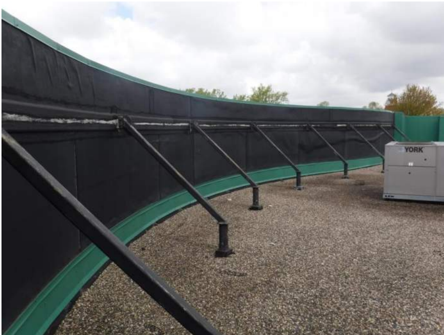
Adhered EPDM membrane cladding on backside of curved parapet of café addition with steel braces
