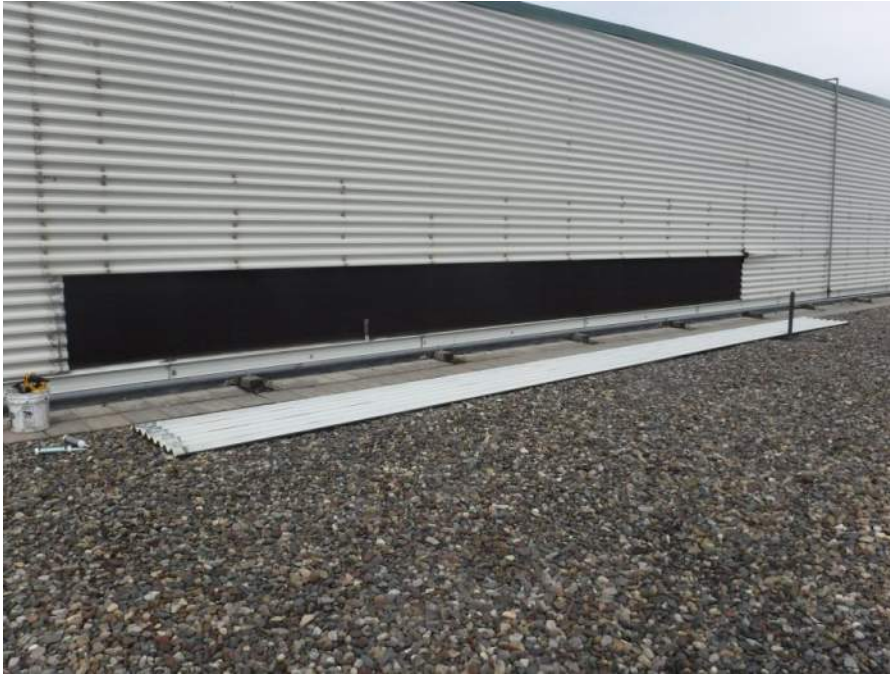
Removed metal panel on east wall of Rink A
