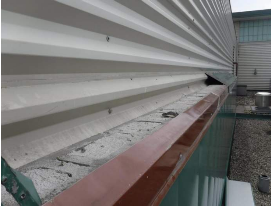
Coping removed from top of CMU wall, coping was sealed to face of corrugated metal panel
