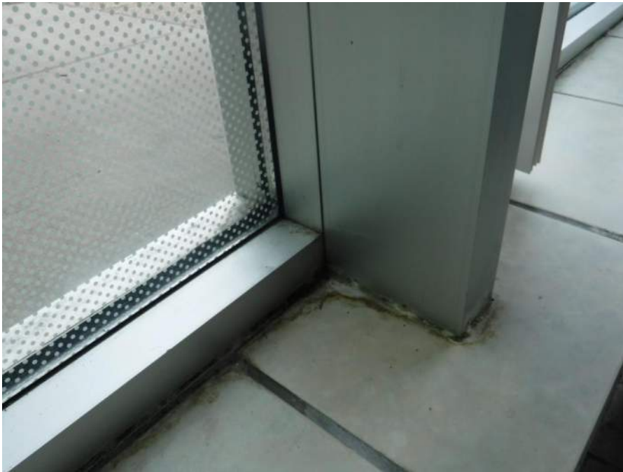
Staining at base of glazing system, note vertical aluminum tube providing reinforcement of store front verticals
