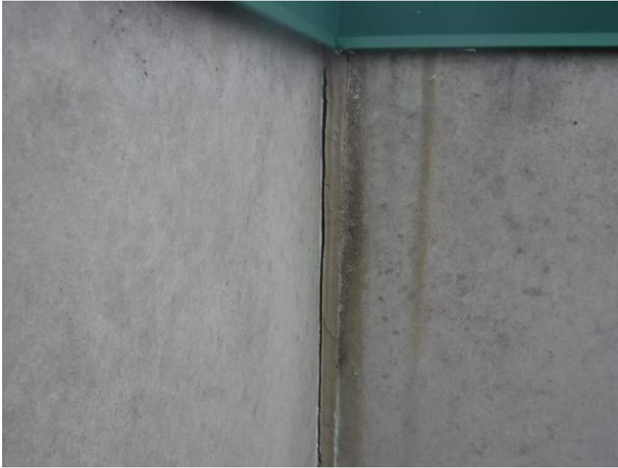
Typical failed vertical sealant joint between precast panels and discoloration
