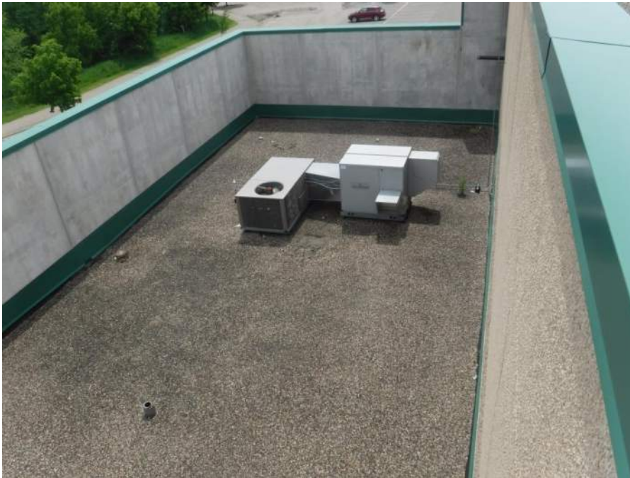
South lower roof east of Rink C, note sample core insulation was saturated
