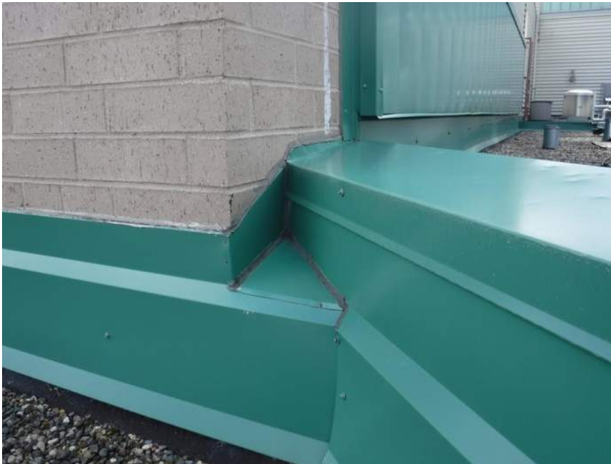
Coping termination to adjacent masonry wall with little upturn and no thru-wall flashing above
