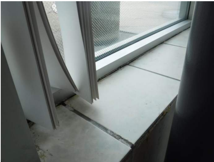
Staining at base of glazing system
