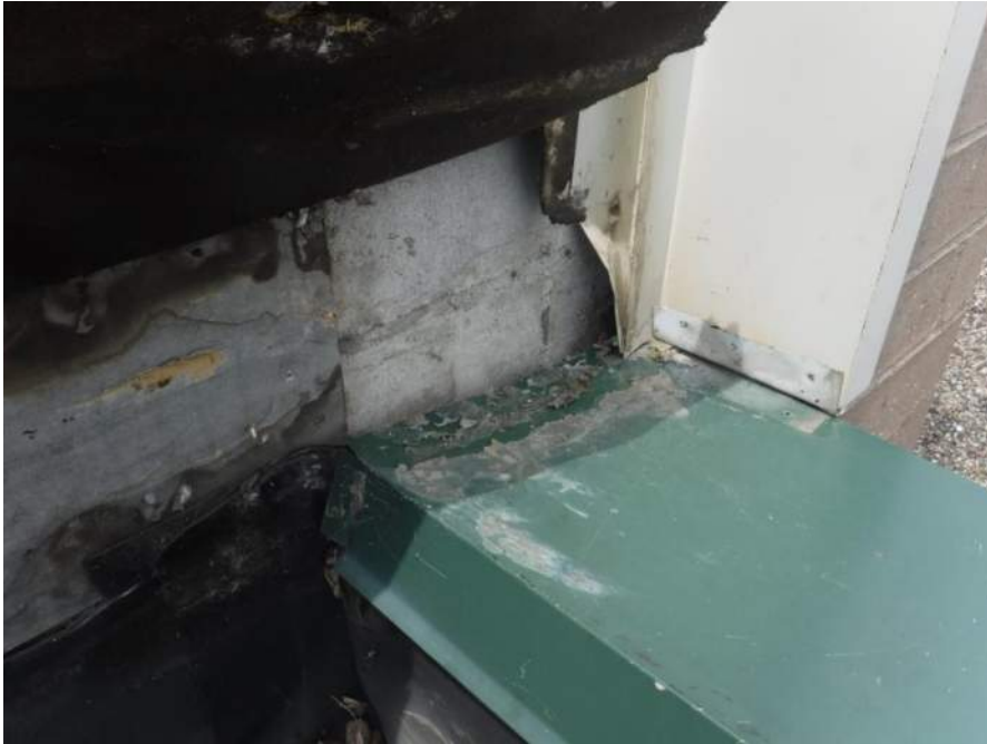
Test opening of previous photo, note membrane and metal does not extend onto adjacent wall at critical interface
