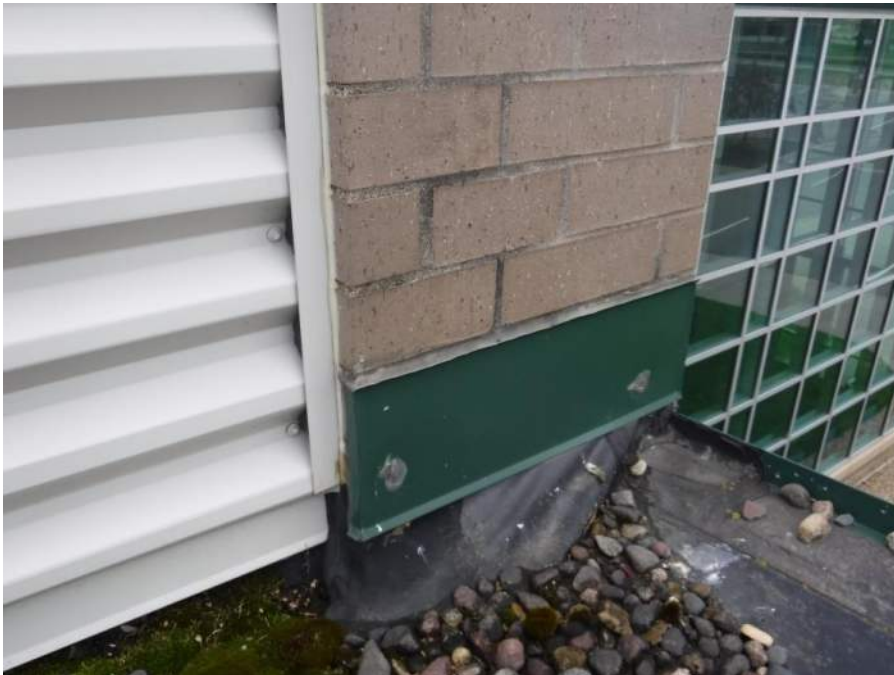
Close-up of previous photo, no masonry thru-wall flashing above the roof termination
