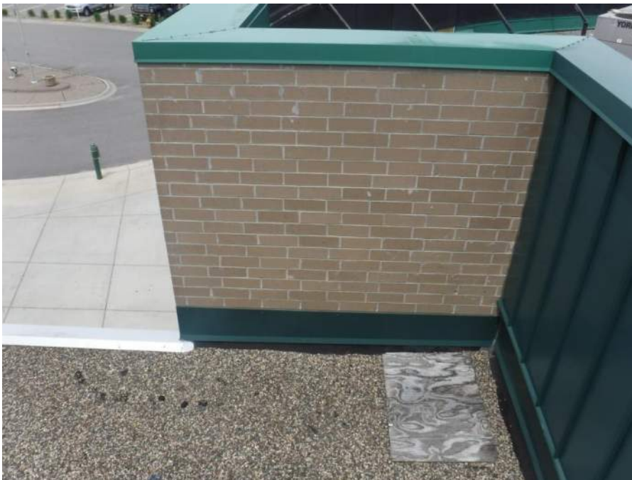
Roof termination to masonry veneer wall at northeast edge of entrance roof with no thru-wall flashing above
