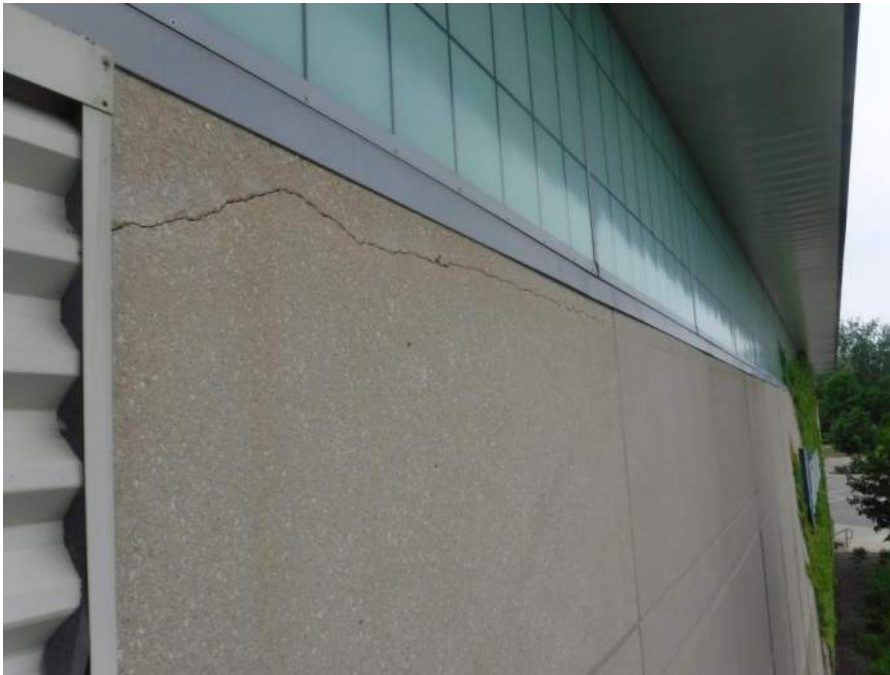
Horizontal crack underneath Rink A clearstory translucent panel
