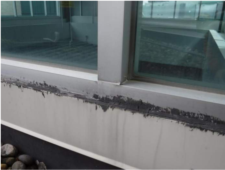
Close-up of window sill, note sealant at horizontal-to-vertical joint, majority of sealant has failed
