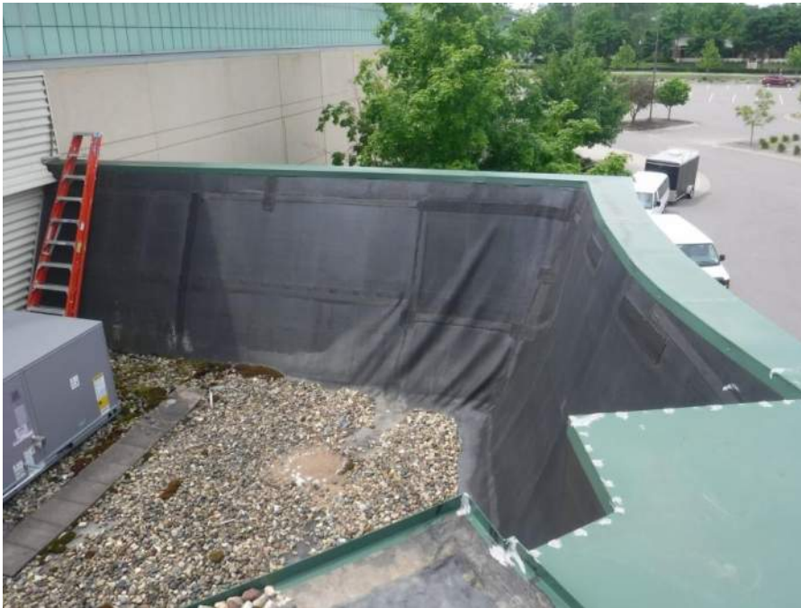
Unadhered membrane at back of sloped parapet west of entrance
