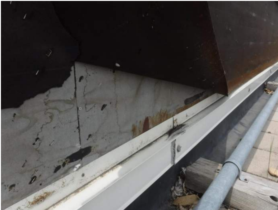
Roof membrane upturn is concealed behind metal flashing which felt paper shingle-laps onto, staining on gypsum sheathing indicates presence of moisture behind felt paper WRB
