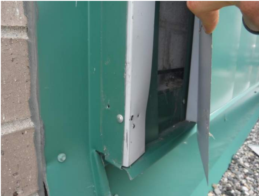
Roof membrane is terminated to face of CMU wall
