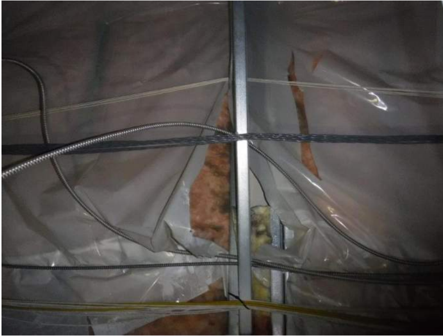
Ineffective vapor retarder on wall between conference room and Rink A, note discoloration on batt insulation
