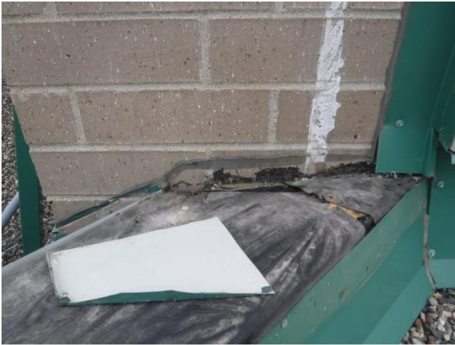
Test opening of previous photo, note lack of upturn and void in membrane flashing
