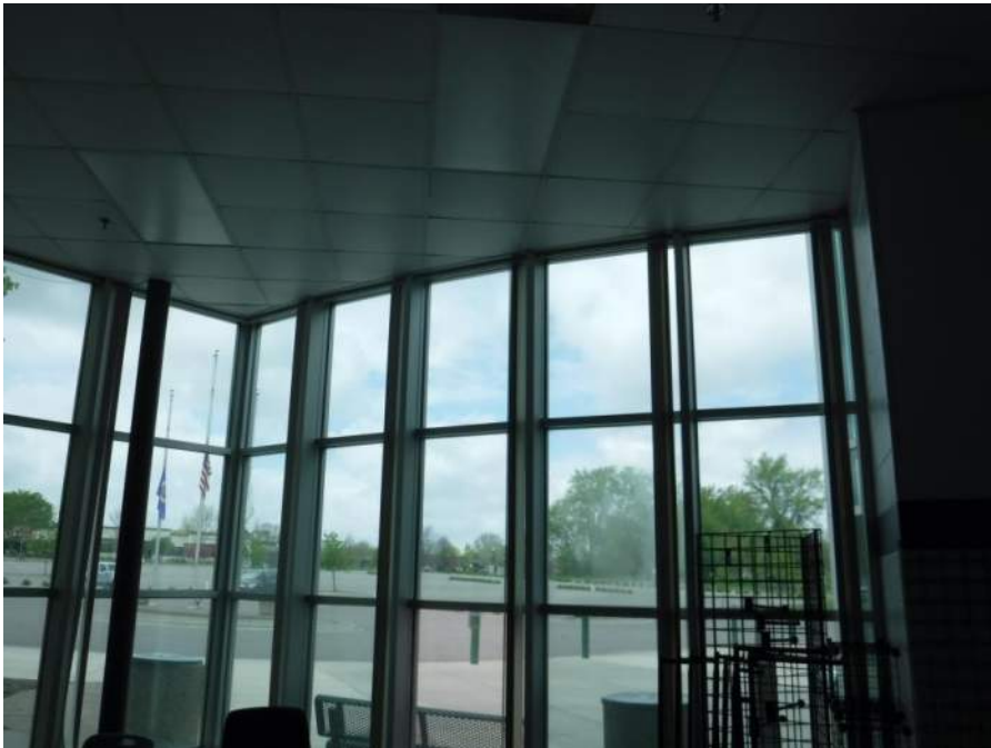
Full-height glazing system in room west of entrance
