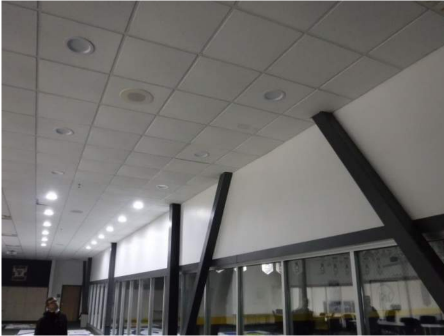
Stained ceiling tiles along wall between conference room and Rink A
