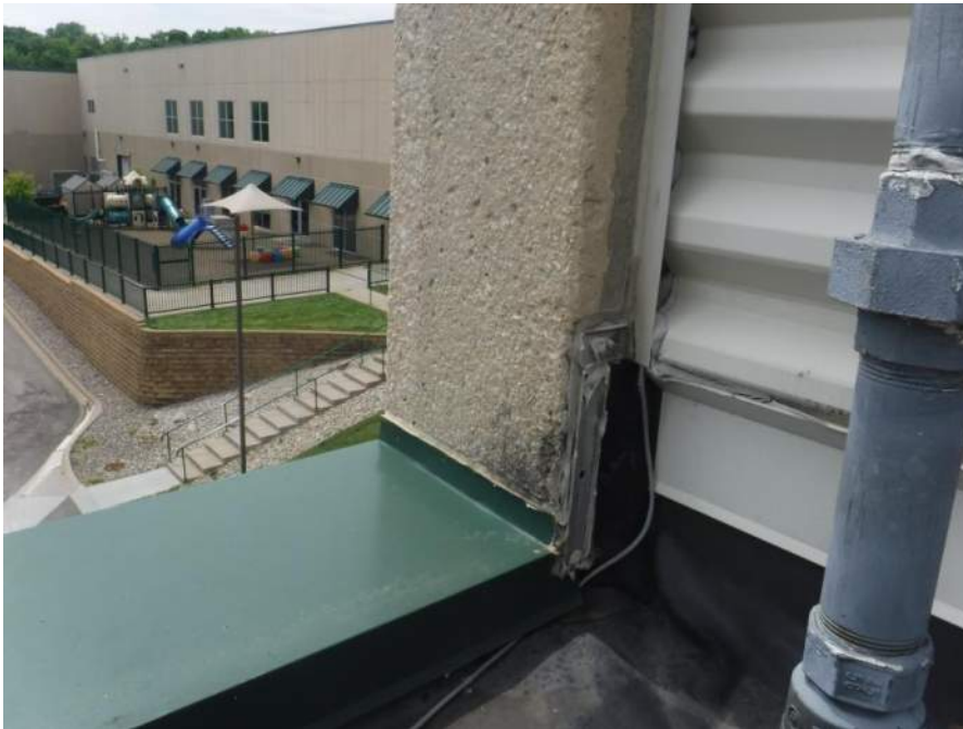
Coping termination to adjacent precast wall, coping end dam is reliant on sealant for water-tightness
