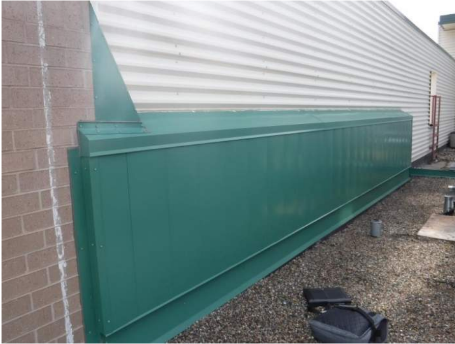
Partial height CMU wall clad with flat-seam metal panel
