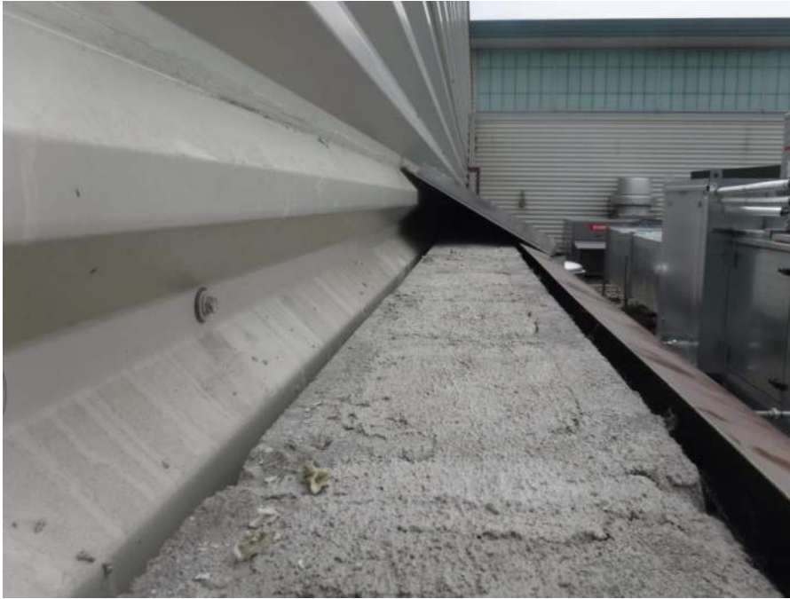
Space between corrugated metal panel and CMU wall is a potential path for water infiltration
