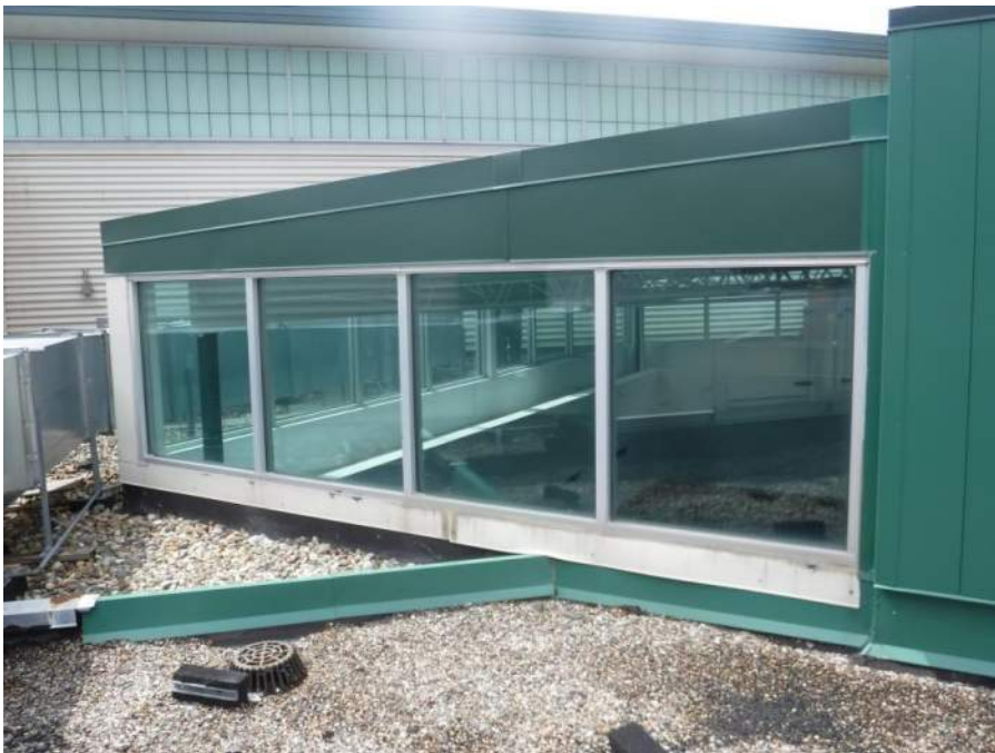
Clearstory windows on northeast elevation of entrance roof
