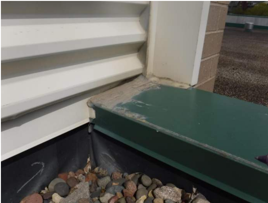
Coping termination to adjacent wall, note sealant applied in attempt to address leak
