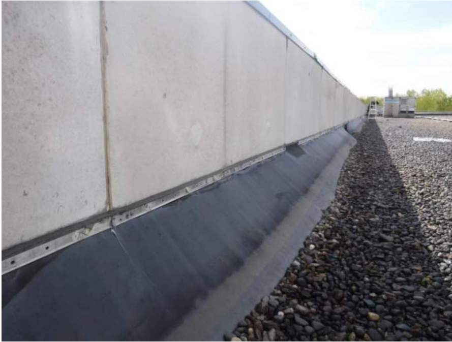
Typical “tenting” observed along ballasted roof perimeters
