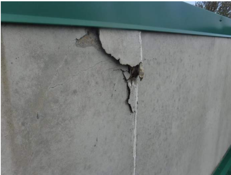
Observed spall in precast, typically caused by presence of moisture and freeze-thaw cycling
