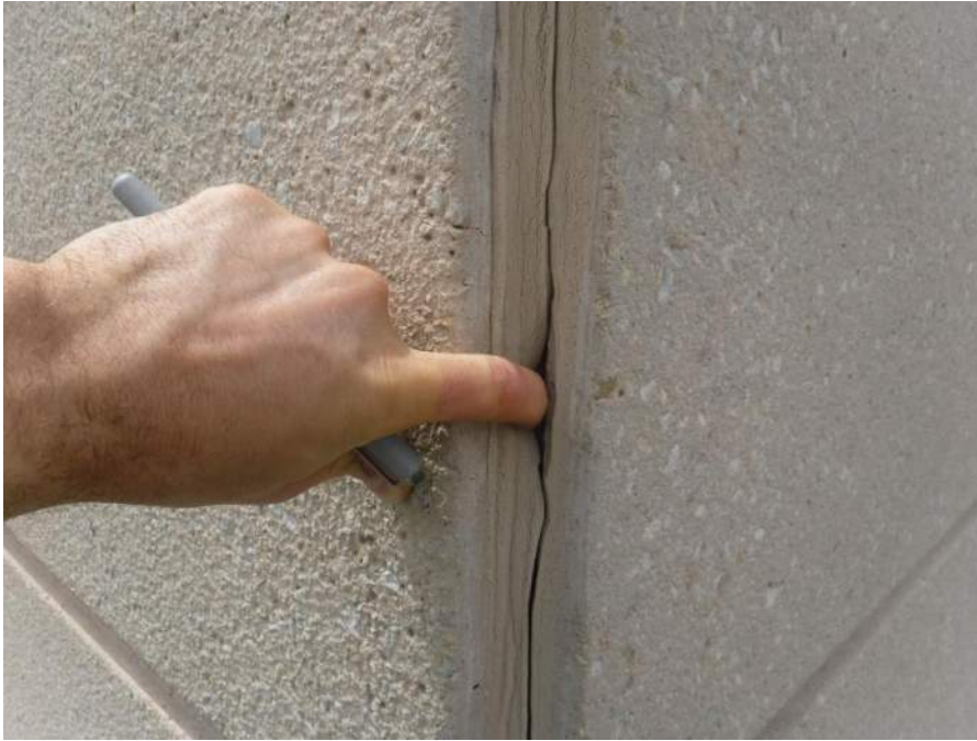
Failed sealant joint at precast outside corner
