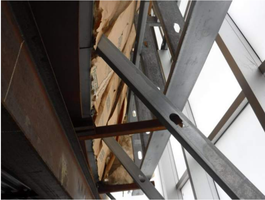
Existing conditions underneath sloped parapet, note staining on kraft-faced batt insulation
