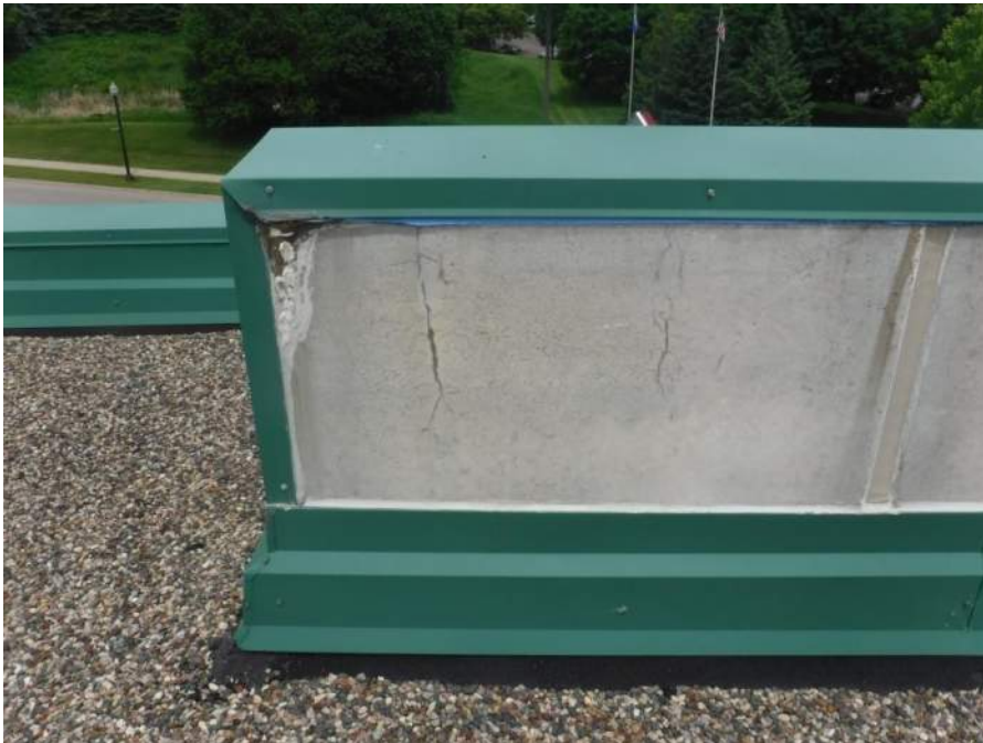
Excessive sealant applied to damaged precast corner and typical hairline cracks
