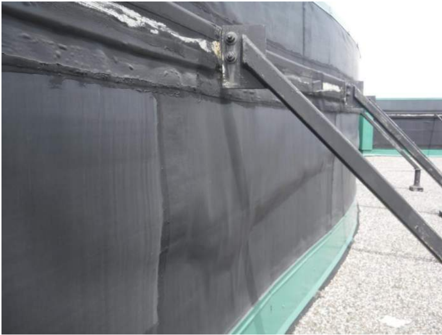
Typical unadhered EPDM membrane
