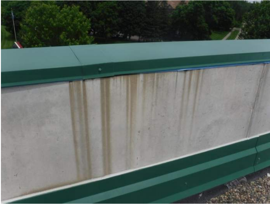
Typical staining originates from beneath coping
