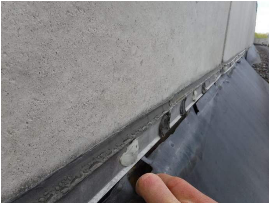
Typical holes in membrane below termination bar caused by “tenting”
