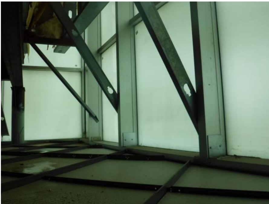
Existing conditions above ceiling, note standing water on ceiling tiles
