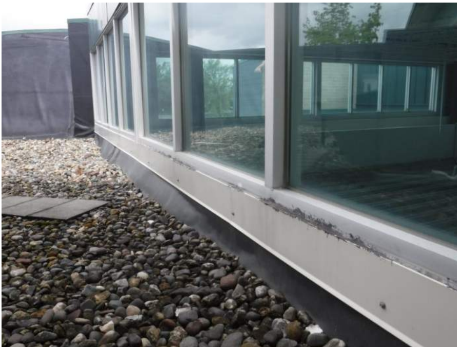
Note different types of sealant applied to joint below sill
