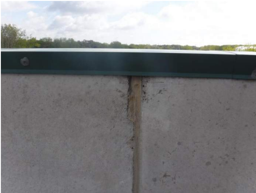
Typical failed vertical sealant joint between precast panels
