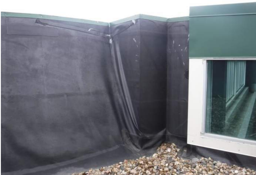
Unadhered membrane at back of sloped and vertical parapet west of entrance
