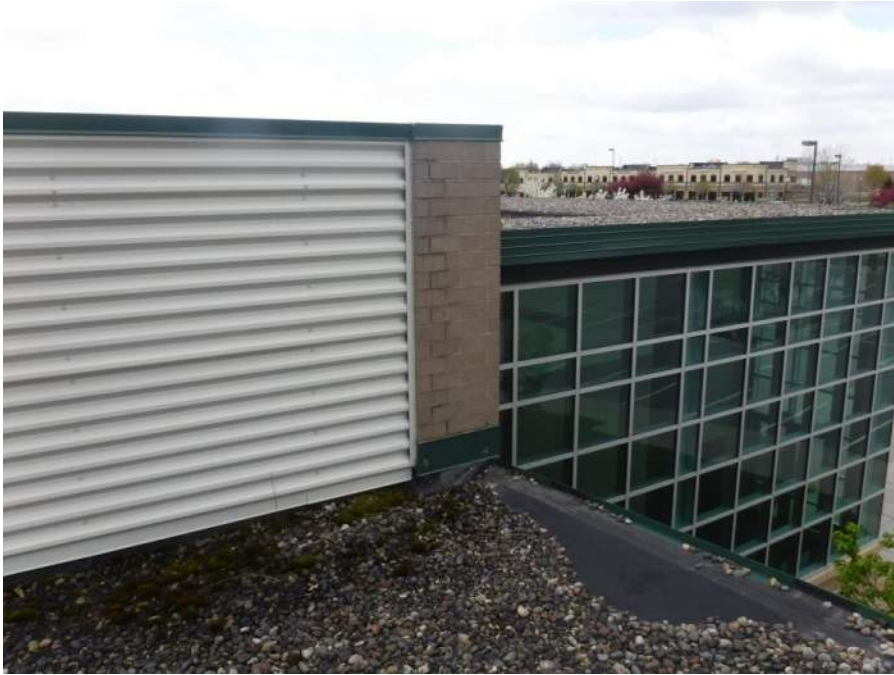
Roof terminated to face of masonry veneer wall return at Rink A southwest penthouse
