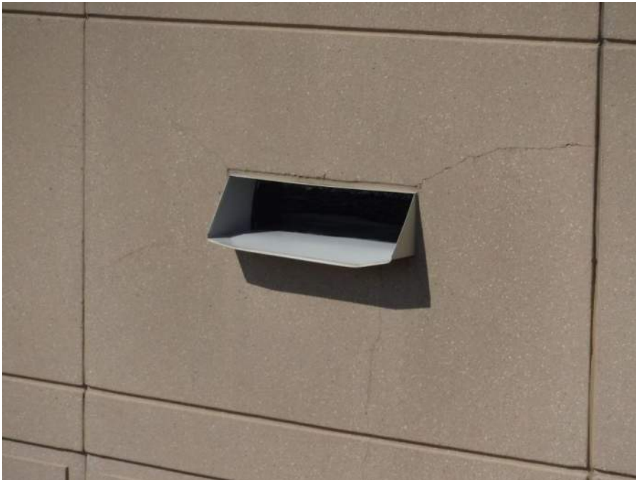
Diagonal cracks originating at corners of scupper penetration
