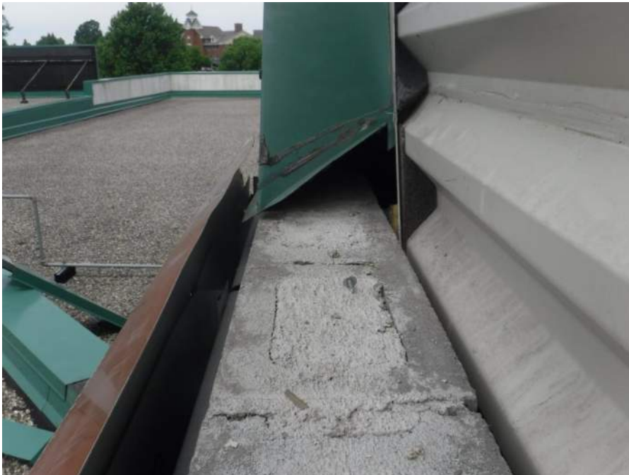
Coping was also sealed to face of adjacent sloped metal panel
