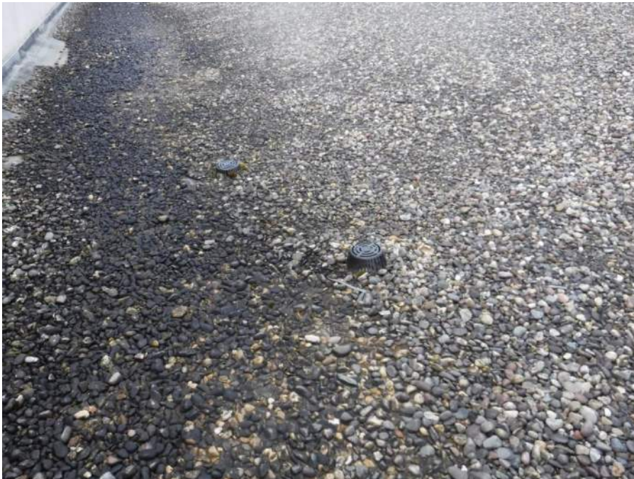
Rink A primary roof drain at higher elevation than standing water
