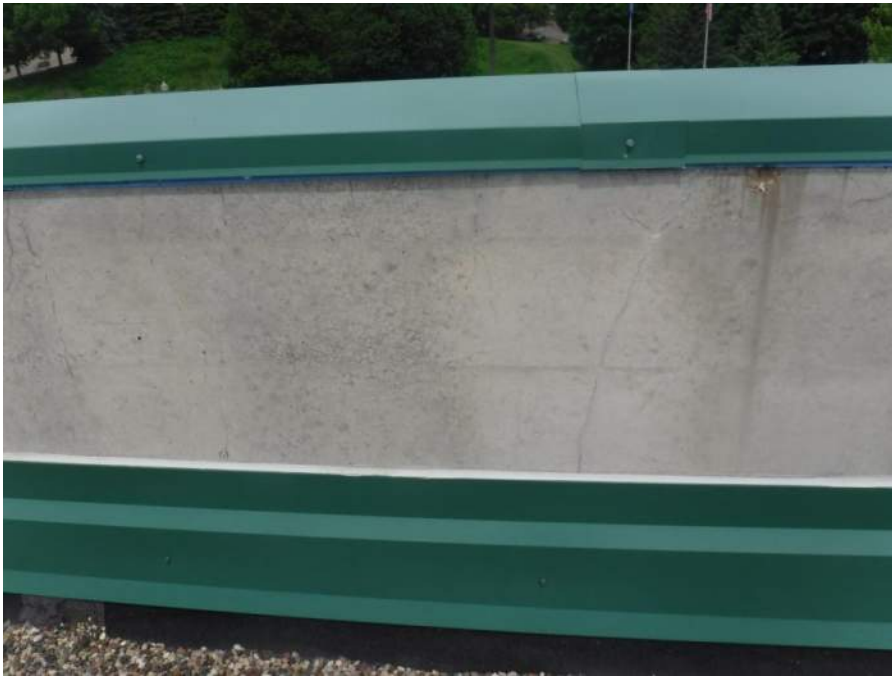
Typical hairline cracks in precast panel
