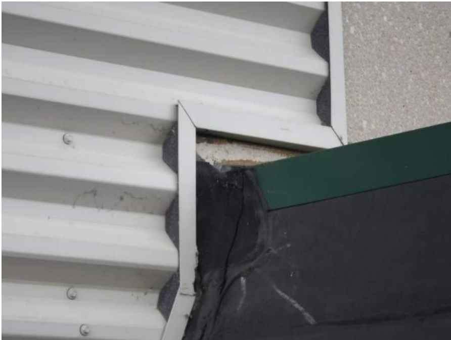
Coping termination to adjacent precast wall with no upturn of membrane or metal coping
