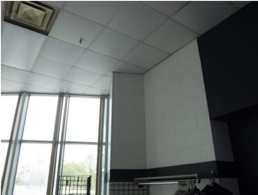
Staining below ceiling observed on CMU wall adjacent to glazing
