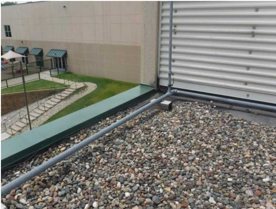
Typical coping with little to no slope
