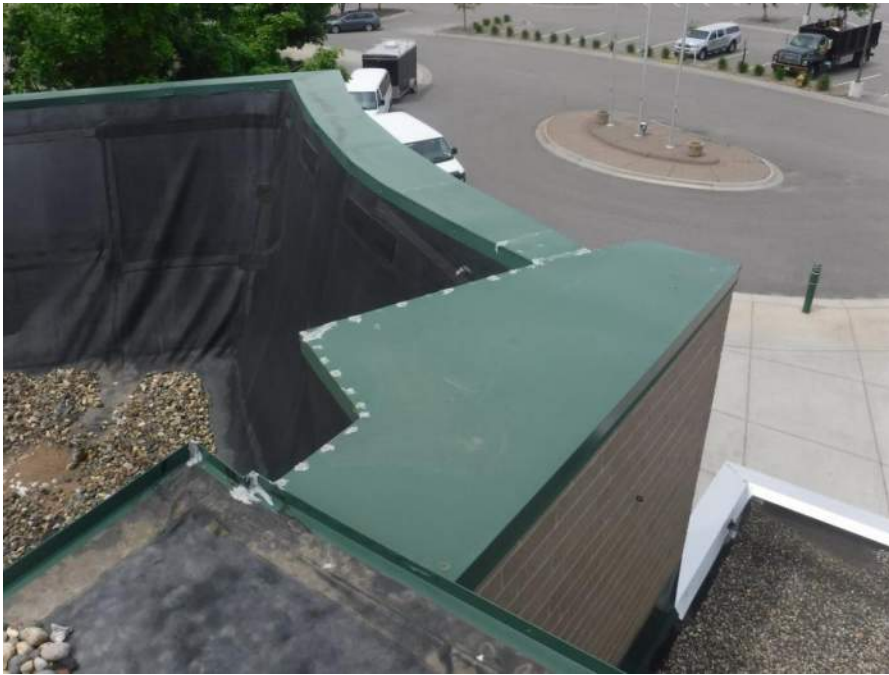
Wide coping west of entrance with little to no slope
