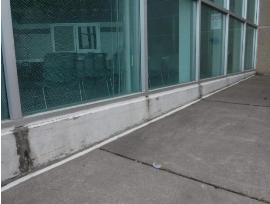
Exterior sill condition, note sealant joint between sill and curb is discontinuous at verticals and staining below verticals
