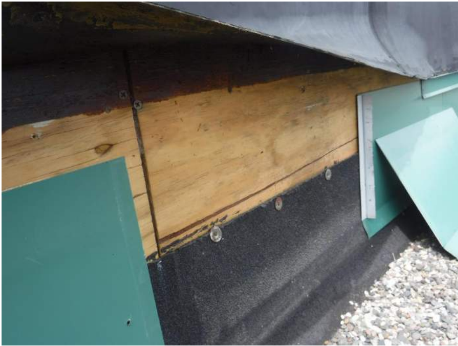
Test opening at base of EPDM clad parapet
