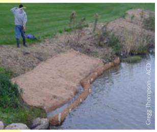
Cococut fiber rolls are a "soft armor" erosion control structure that is effective in areas of low to moderate shoreland erosion. It is a dense "log" of coconut fiber wapped in a coarse jute net and /or burlap. They come in 8", 12" and 20" diameter rolls. When a roll is secured along the toe of an
